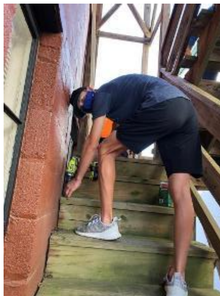
Making repairs to the fire escape.
